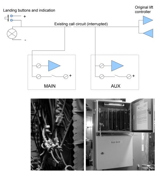
The call splitter panels have been mounted on the end of the existing 'Progressive Logic' controller. The existing call circuits has been cut, numbered, and tied off (light wires). Black wires have been crimp connected onto each end and go to the MAIN or AUX splitter panels. The MAIN panel is open (above) and has 2 calls latched, ie 2 relay LEDs showing.
